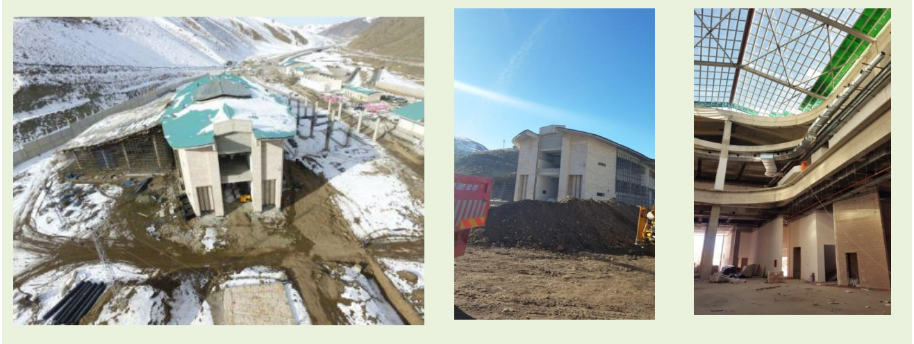
Figure 17. Construction of Kapiköy Checkpoint
