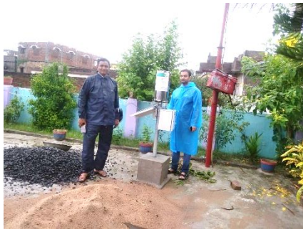
Inspection of telemetric weather station in Bihar.
