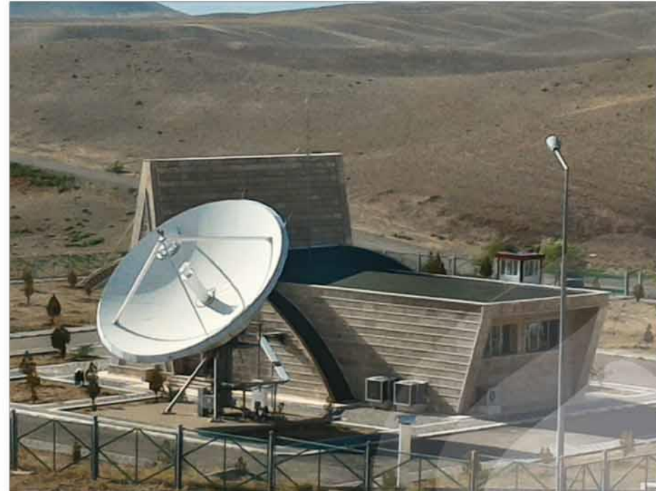
Back-up Satellite Ground Control Station in Nakhichevan Autonomous Republic
