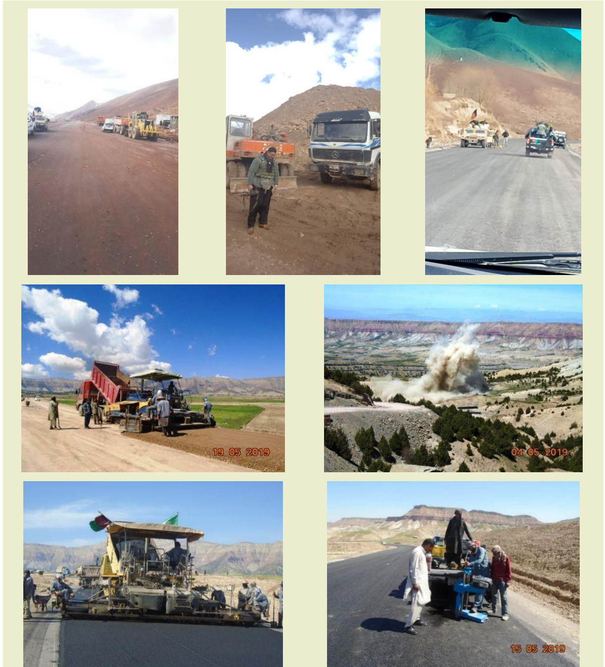
Figure 13. Construction of 80 km road after Herat
