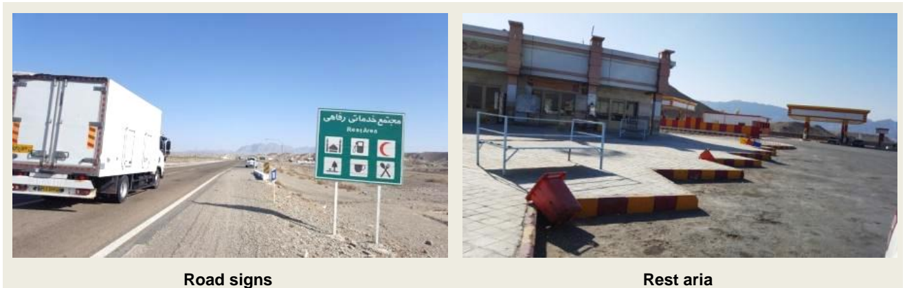
Figure 16. Photos of road monitoring Chabahar - Zahedan (IRN)
