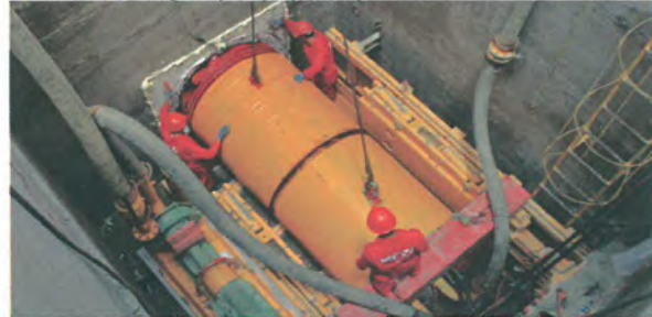
▼ Hamedan Sewerage Project by Pipejacking Method, Iran
