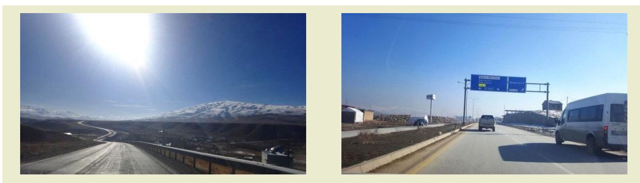
Figure 12. Photos of road monitoring Van – Esendere (Turkey)
