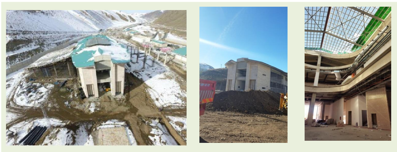
Figure 17. Construction of Kapiköy Checkpoint
